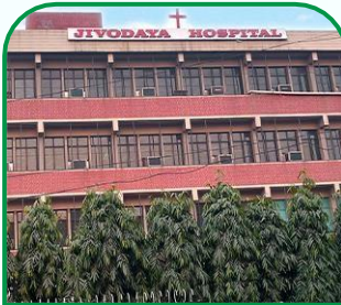
Jivodaya Hospital, Ashok Nagar, Delhi
