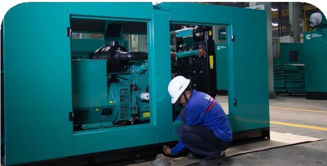
DG & Repair Maintenance
